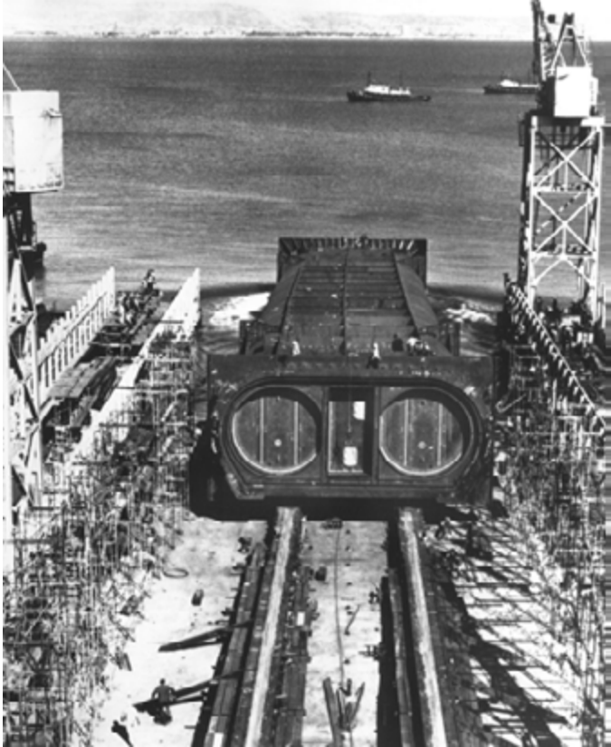
Part of the Transbay Teriminal being lowered into the Bay, courtesy of Bay Area Rapid Transit
